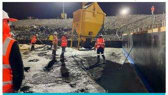
The project achieved a significant milestone on 9 September with the first concrete poured for the weir. Over the next 12 months more than 100,000m<sup>3</sup> of concrete will be poured and over that time the weir will begin to rise from the river bed.
