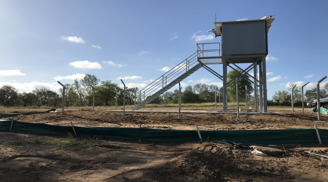
The Fitzroy River has a new gauging station located 10km downstream from the weir at Hanrahan Crossing. The station will monitor environmental flow releases and water supply releases from the weir and will help build the overall understanding of the river hydrology for decades of future planning and weir operations to come.
