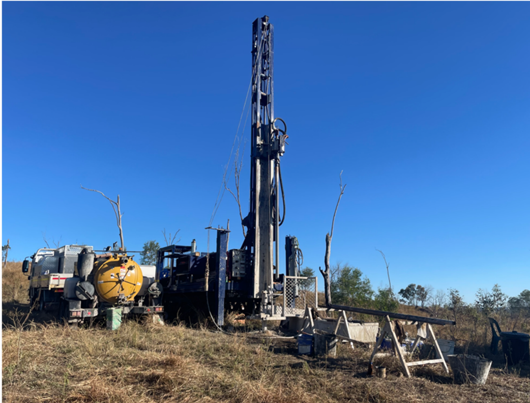
Figure 8: Investigatory drilling site set-up and equipment
