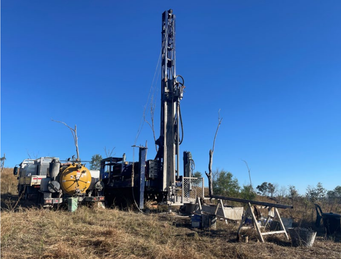
Figure 8: Investigatory drilling site set-up and equipment
