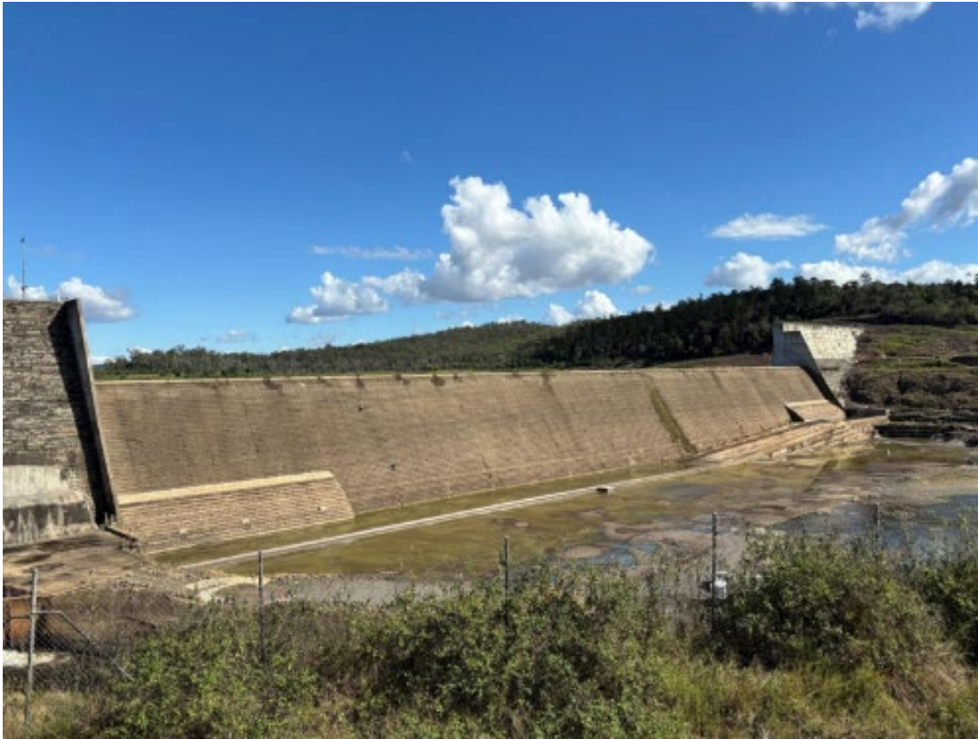
Figure 1: Lowered Paradise Dam wall (Source: Paradise Alliance 2025)
