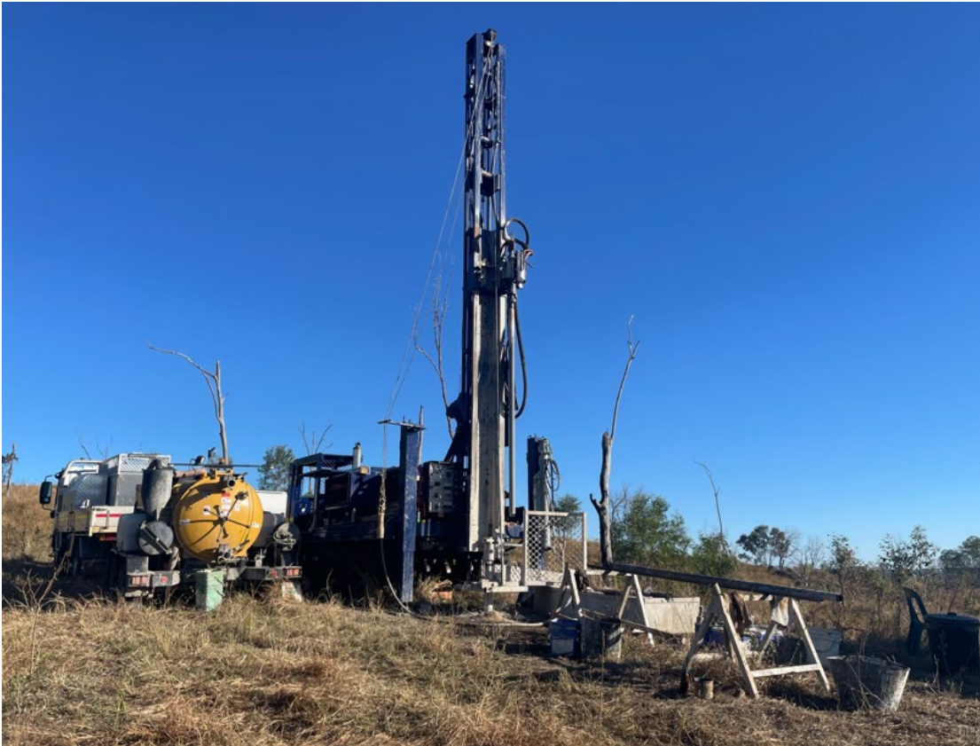
Figure 8: Investigatory drilling site set-up and equipment
