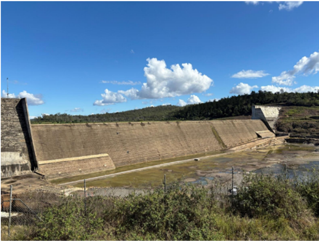
Figure 1: Lowered Paradise Dam wall (Source: Paradise Alliance 2025)
