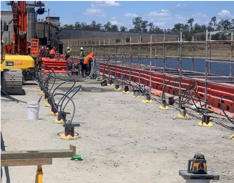
Figure 1: Rows of passive anchors installed and ready for grout fill
