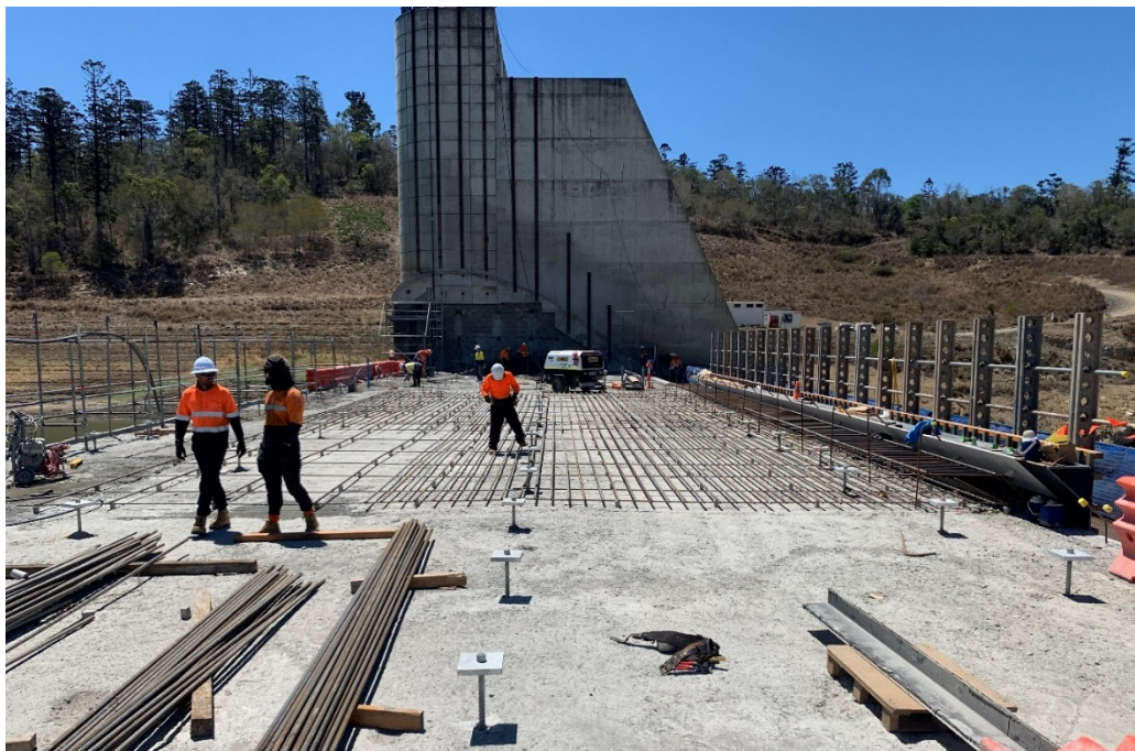
Figure 1: Steel reinforcement in preparation for concrete pours to construct the new crest
