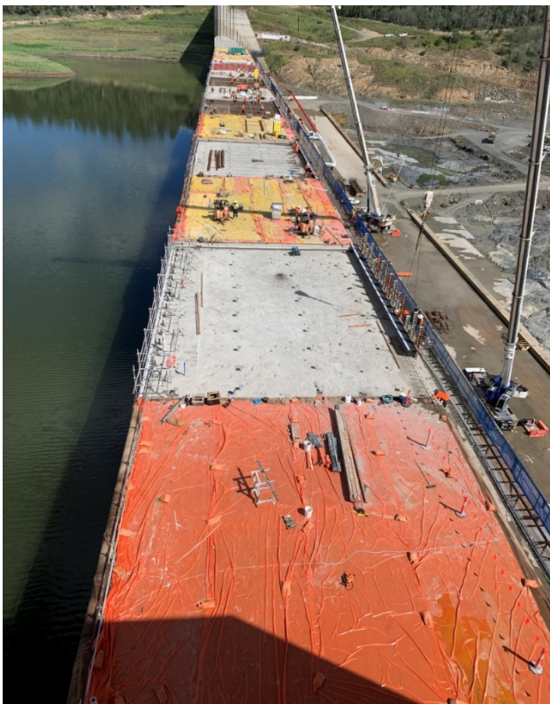
Figure 1: Construction activity for the new concrete crest
