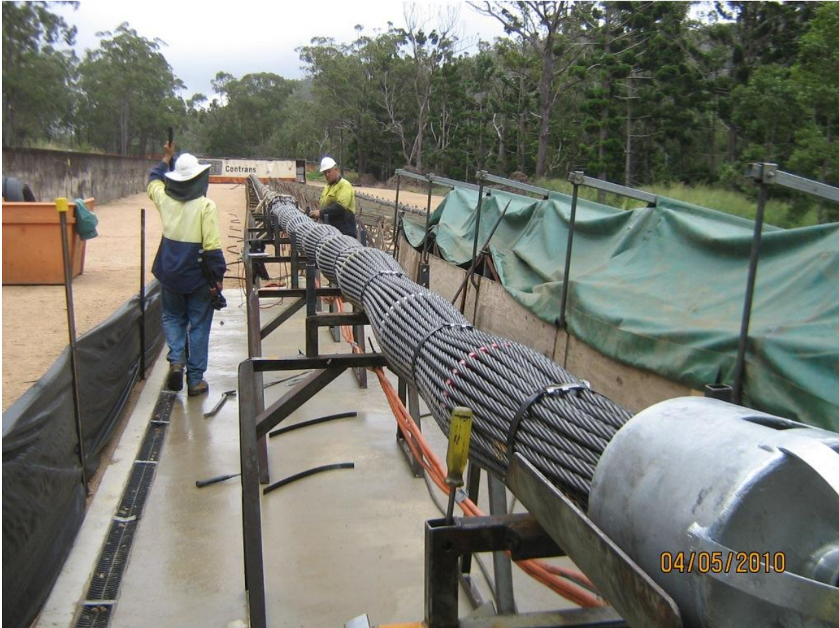
Figure 1 - 75 Strand anchor ready for installation at Tinaroo Falls Dam
