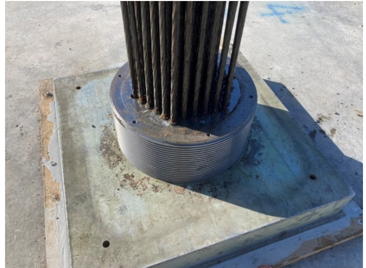
Figure 5 – Locked-off anchor following stressing.
