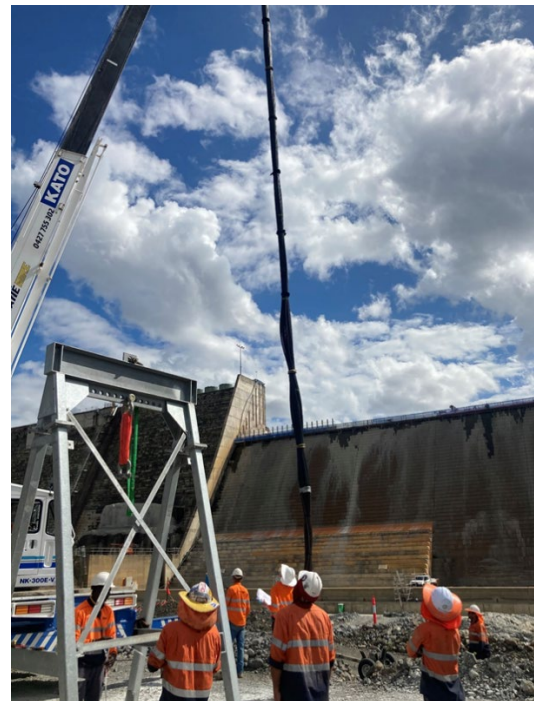
Figure 3 – Lifting anchor to lower into vertical borehole.
