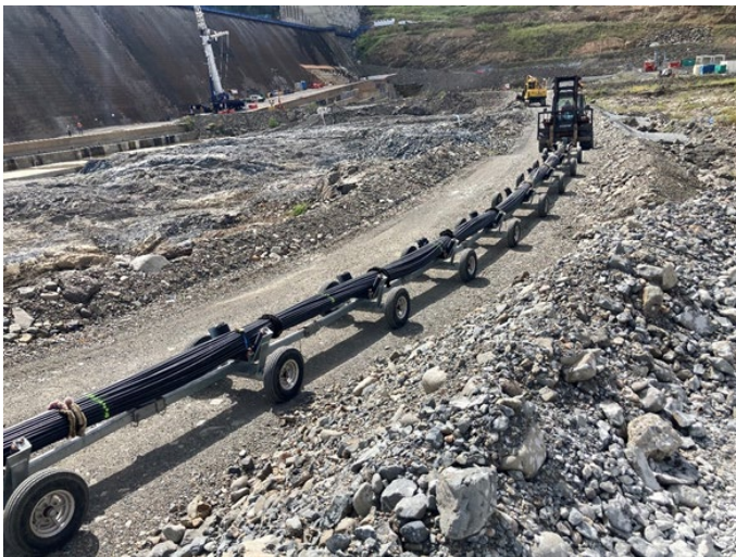
Figure 2 – Transporting a post-tensioned anchor from the fabrication yard to installation site.
