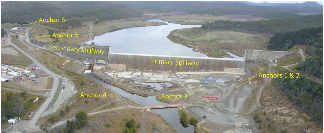
Figure 1 – Anchor trial locations at Paradise Dam.
