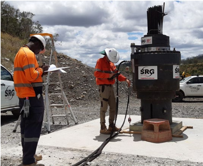
Figure 4 – A 2200 tonne hydraulic jack stressing a 91 strand anchor.
