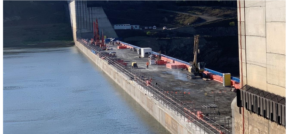
Paradise Dam Essential Works, Bundaberg — complete
