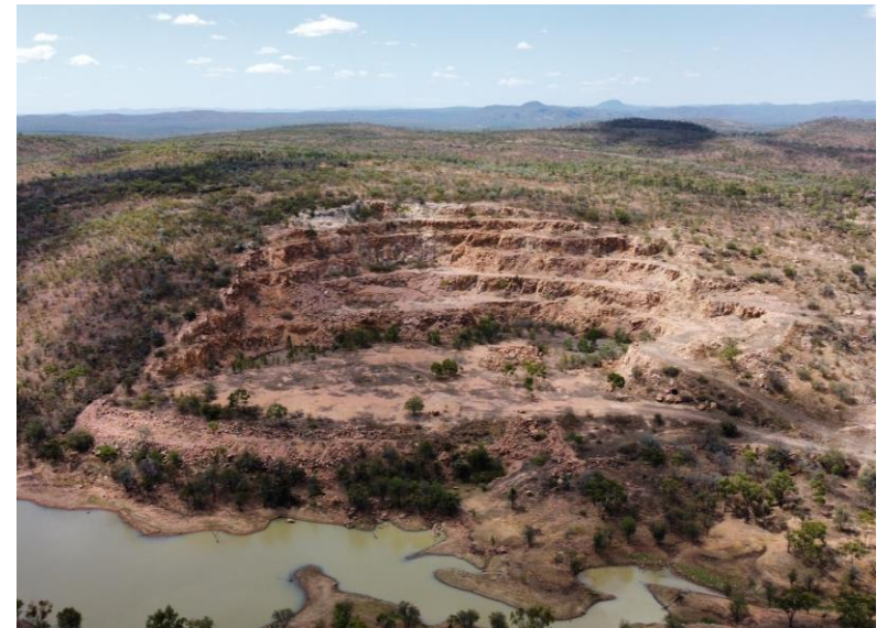
Existing quarry from original construction
