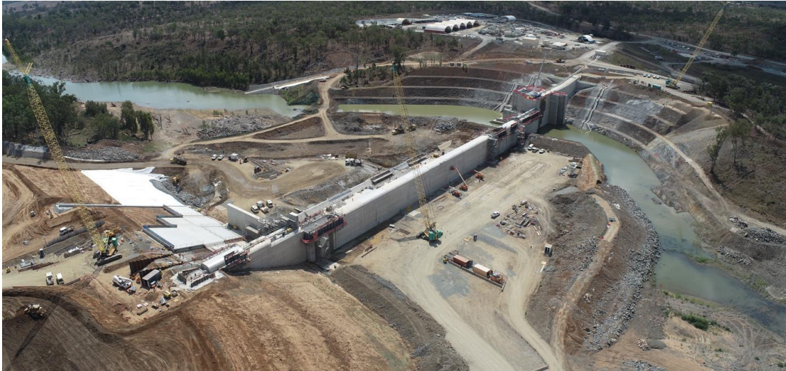
Rookwood Weir Project, Central Queensland — near-complete
