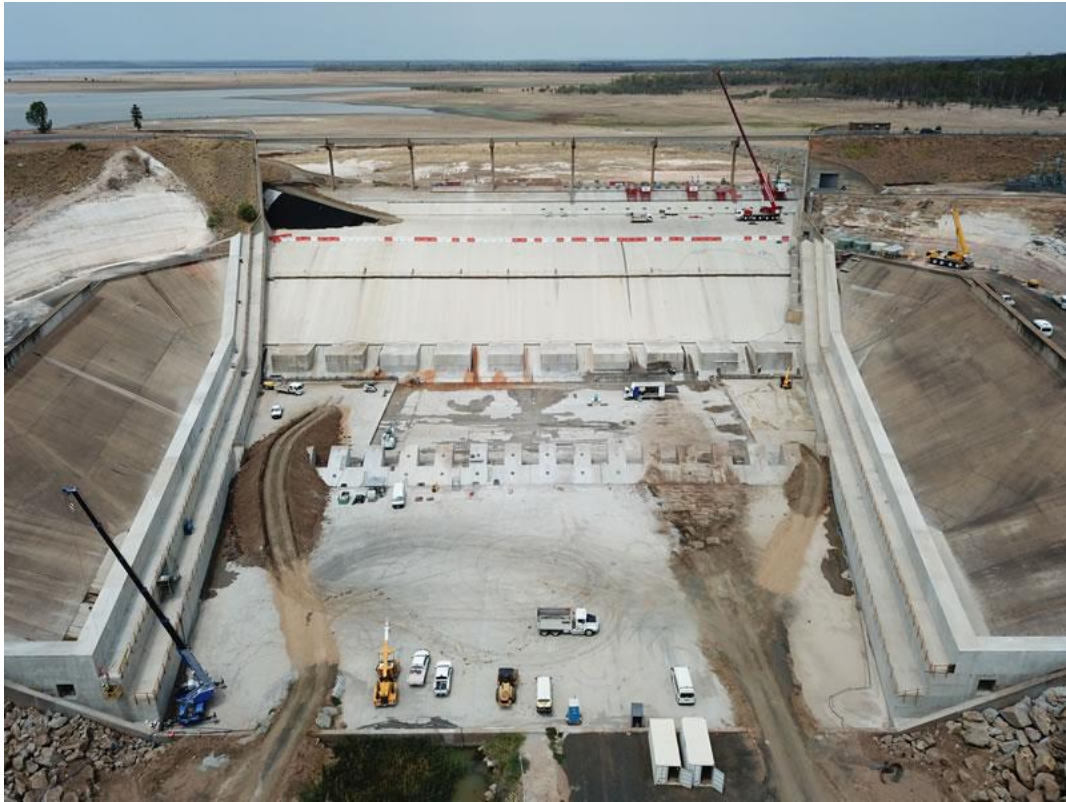
Fairbairn Dam Improvement Project, Emerald — completed 2020
