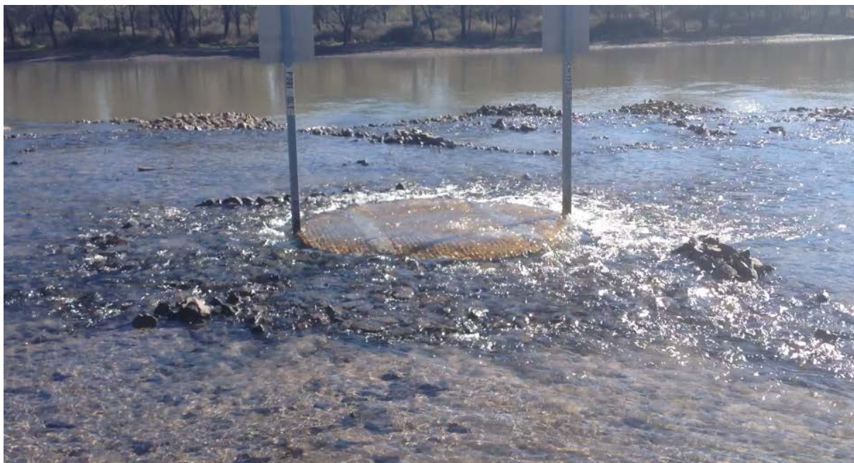
Photo 1: Kenya to Chinchilla Weir Pipeline Outfall
