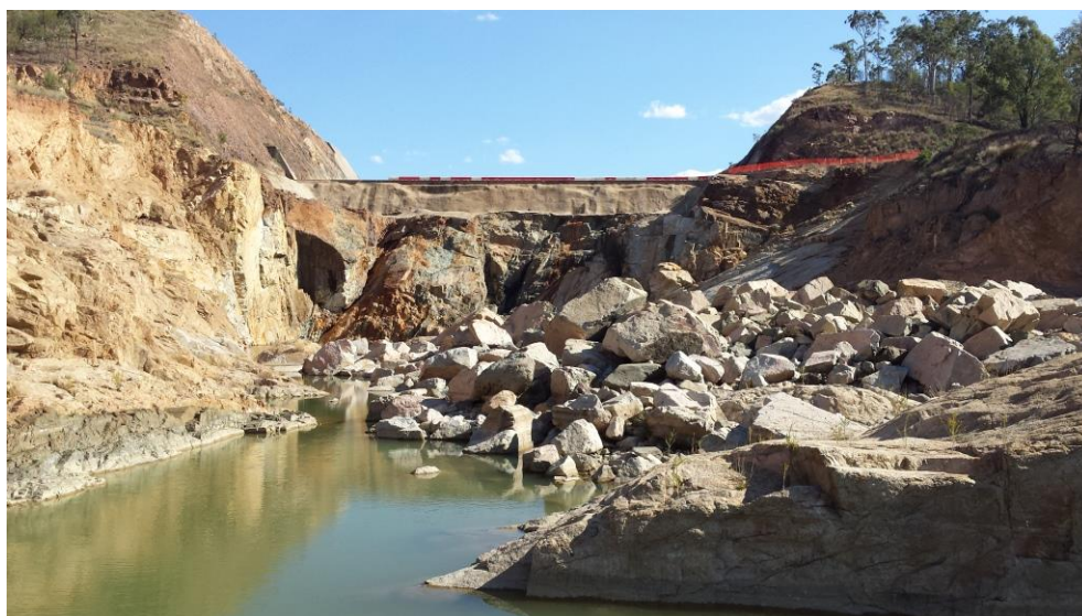
Figure 1.3: Flood damage to the Boondooma Dam spillway, 2013
