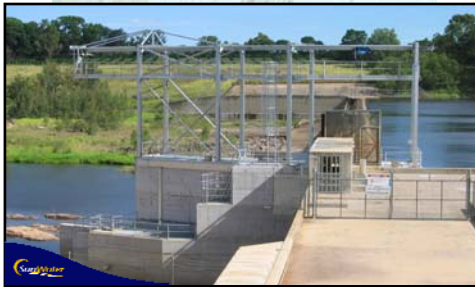
4. Claude Wharton Weir – Fish Lock
