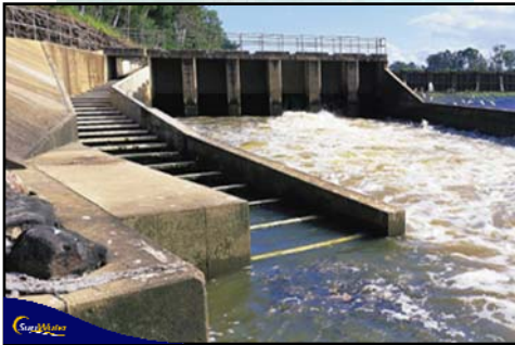
1. Ben Andersen Barrage – Vertical Slot Fishway
