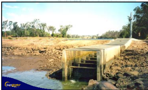
7. Kolan Barrage – Vertical Slot Fishway
