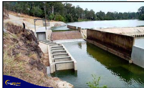
8. Mary River Barrage – Vertical Slot Fishway
