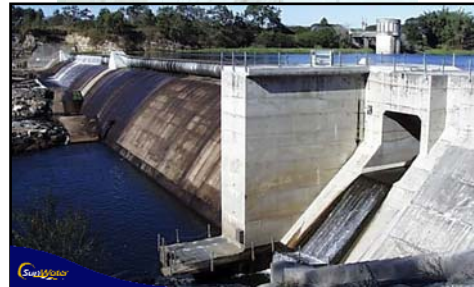
5. Dumbleton Weir – Fish Lock
