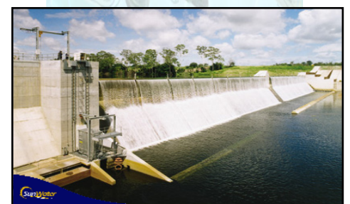
12. Ned Churchward Weir – Fish Lock
