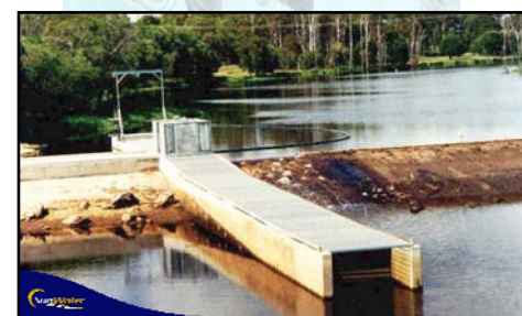
11. Tinana Barrage – Vertical Slot Fishway
