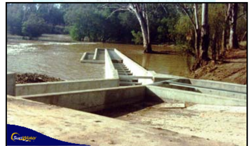
9. Moura Weir – Vertical Slot Fishway
