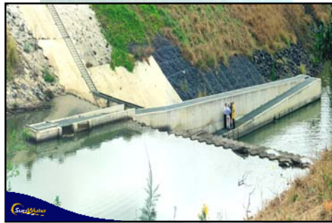
2. Bromelton Weir – Vertical Slot Fishway
