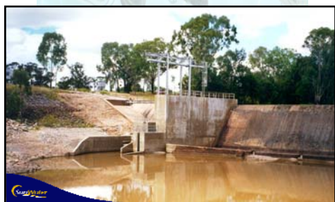
10. Neville Hewitt Weir – Fish Lock
