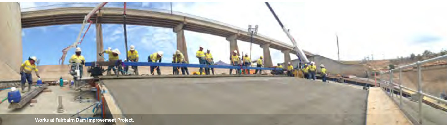
Works at Fairbairn Dam Improvement Project.
