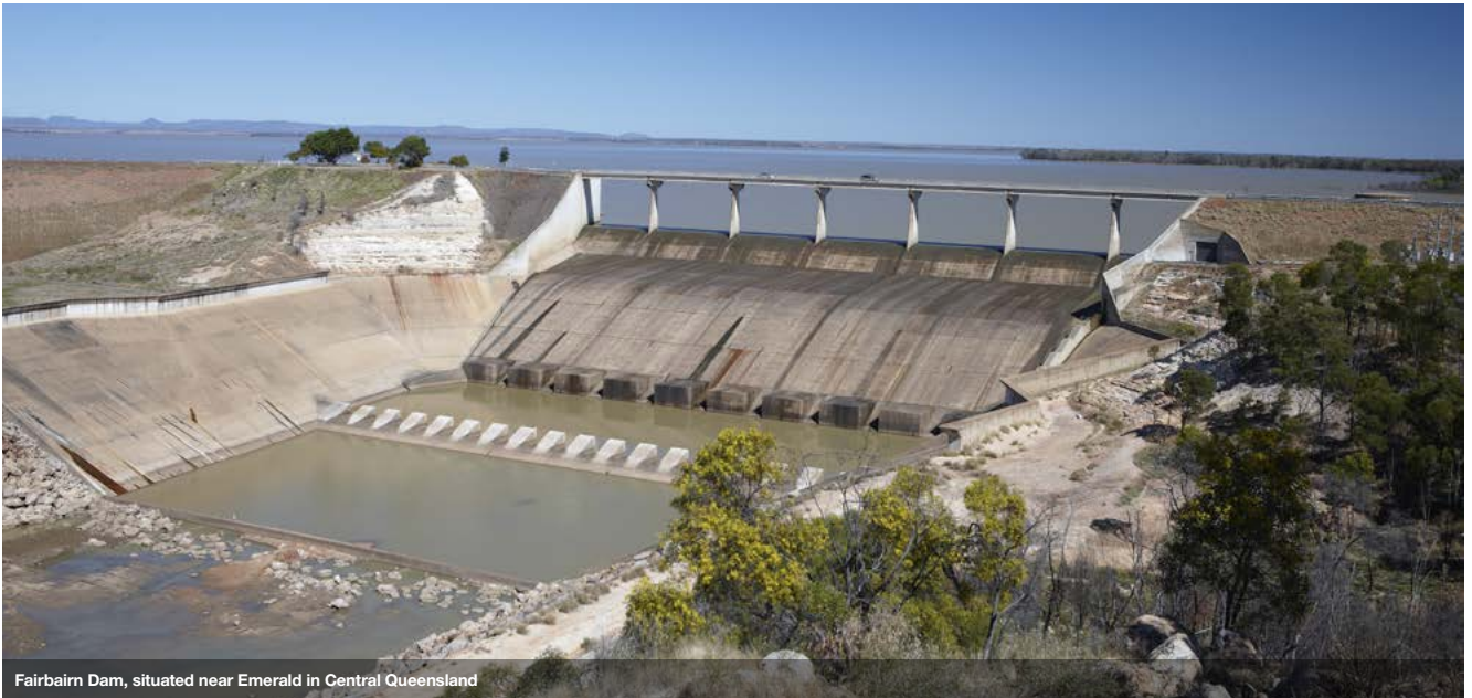
Fairbairn Dam, situated near Emerald in Central Queensland
