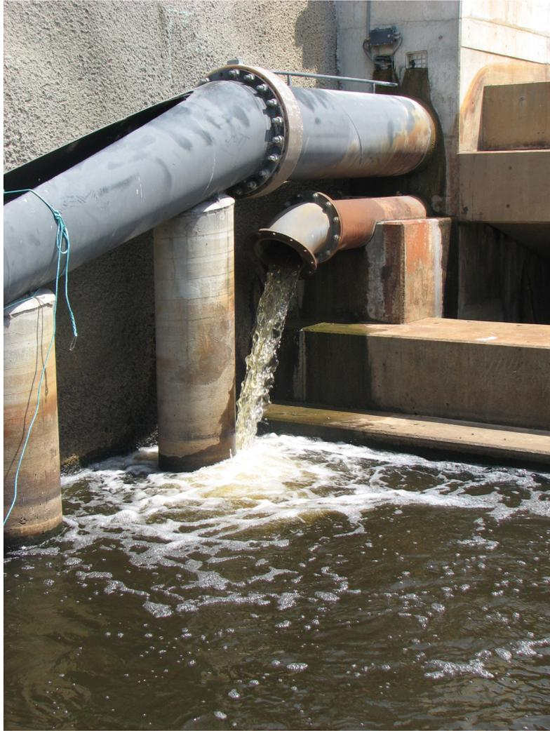
**Figure 24** Downstream fishway outflows during attraction phase in the outlet release channel.
