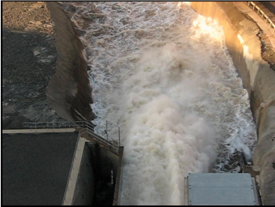
**Figure 18** Flow conditions downstream of the fishway entrance slot during an environmental outlet release of 40 cumecs.
