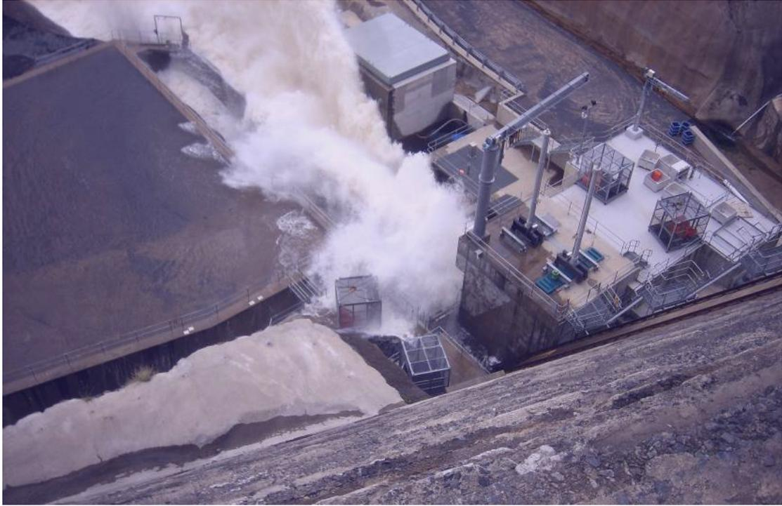
**Figure 20** Flow conditions in the fishway entrance slot during an environmental outlet release of 240 cumecs and 120mm spillway flow 23<sup>rd</sup> September 2010.
