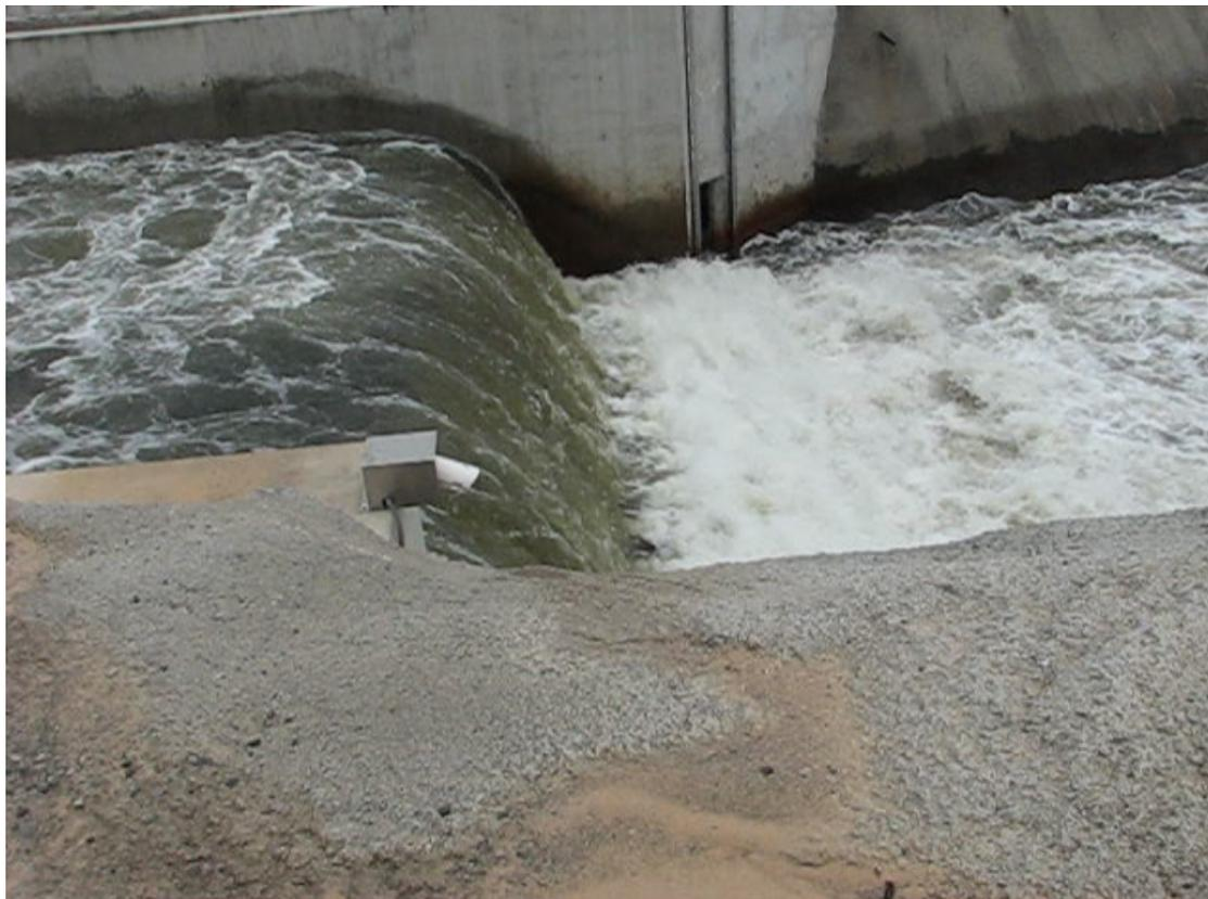
**Figure 17** Flow conditions downstream of the fishway entrance slot during an environmental outlet release of 20 cumecs.
