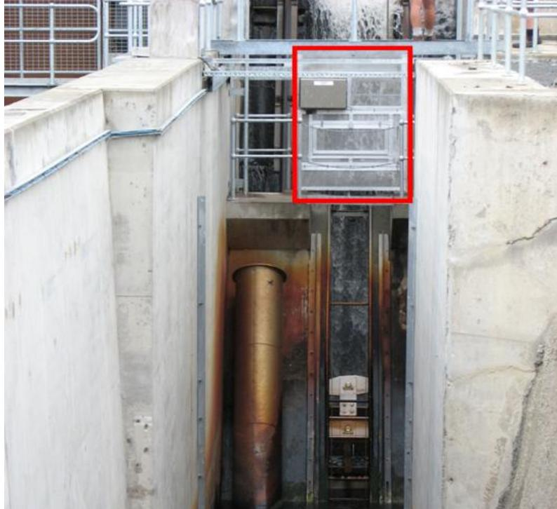
**Figure 23** Quad leaf gate arrangement at the fishlift entrance slot, red outline shows the screen over the gate hoist.
