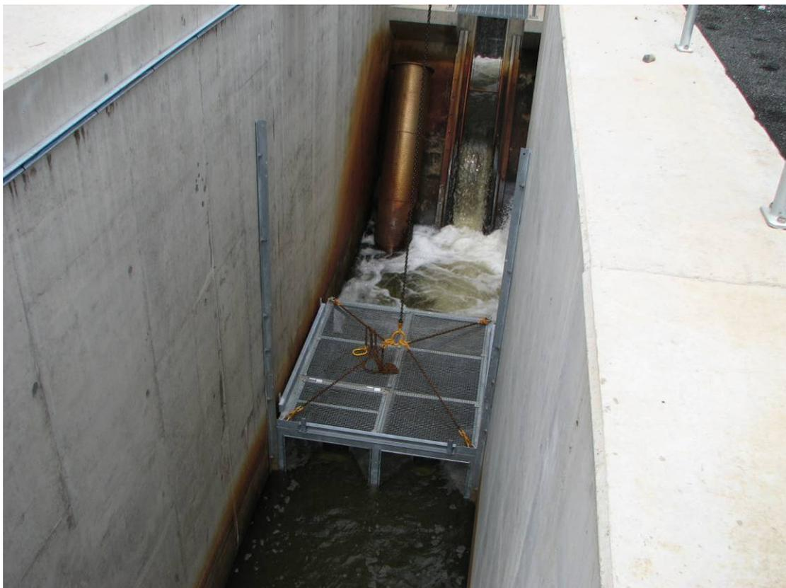
**Figure 5** The upstream trap set in place within the fishlift approach channel.
