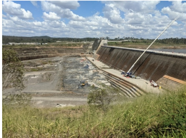
Figure 2 – Preparatory excavation work
