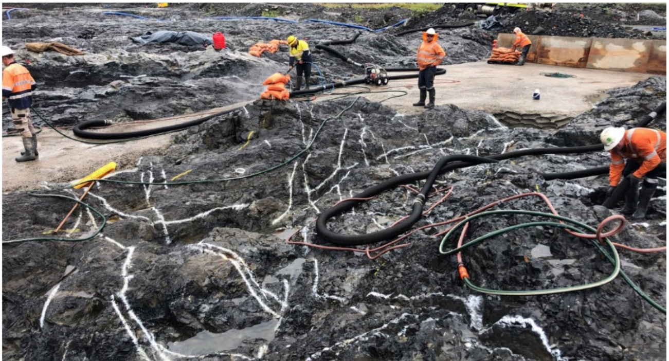
Figure 3 – Rock clean-up for mapping and dental concrete
