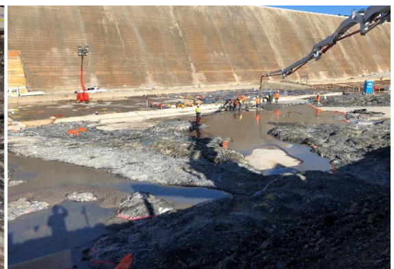
Figure 5 – Dental concrete being placed
