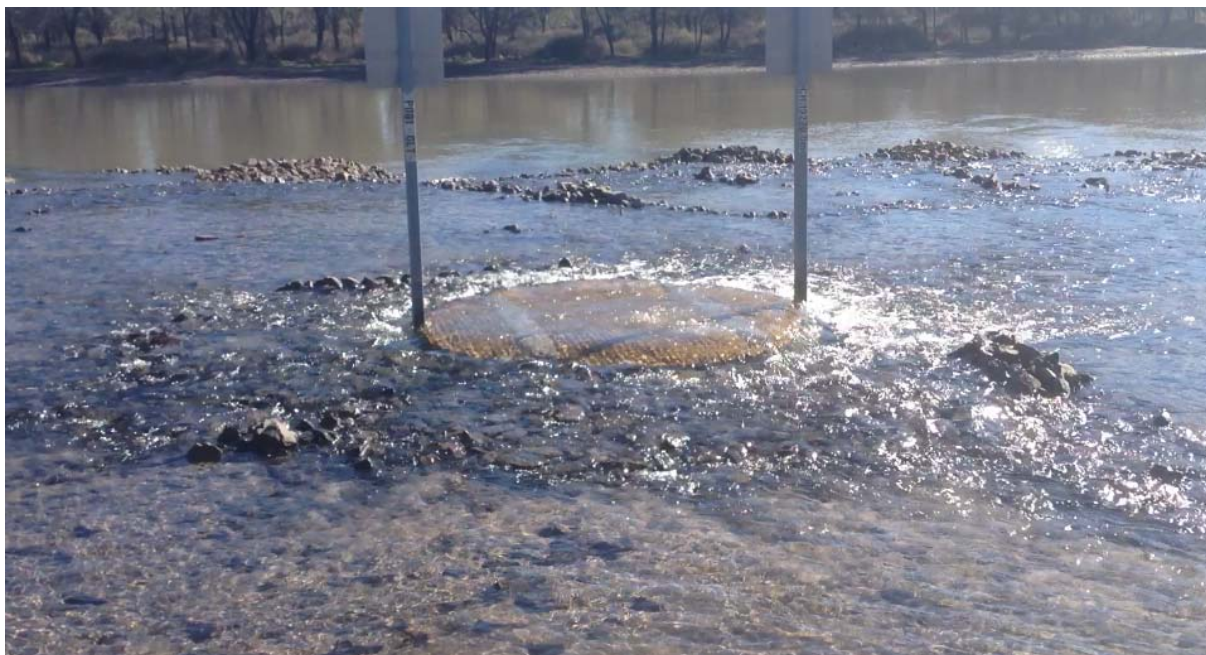
Photo 1: Kenya to Chinchilla Weir Pipeline Outfall
