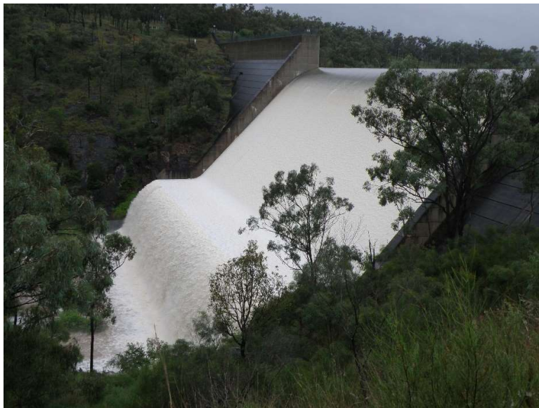
Photo of Wuruma Dam spillway
