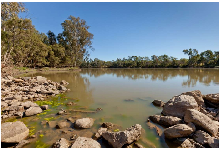
Photo of Neville Hewitt Weir
